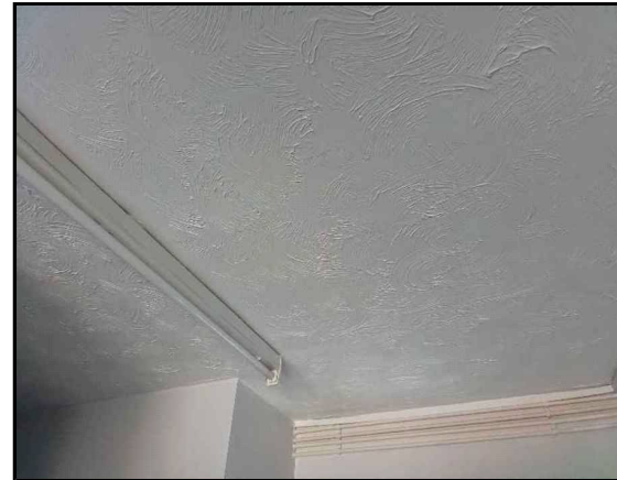
Ground Floor Utility Room (G.002) Textured Coating/Paint Ceiling,
