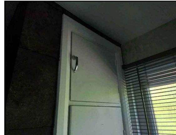
1st Floor Bathroom (1.003) Inaccessible Bulkhead
