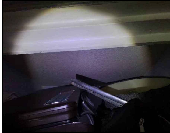
Ground Floor Living Room/Lounge (G.006) Textured Coating/Paint Ceiling, Within cupboards
