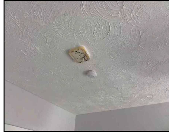
1st Floor Landing (1.007) Textured Coating/Paint Ceiling,
