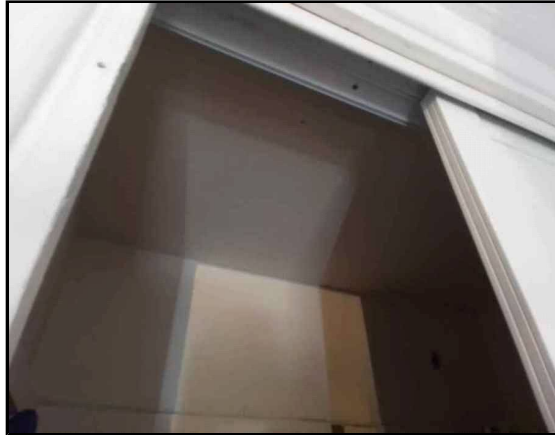
1st Floor Bedroom 4 (1.006) Textured Coating/Paint Ceiling, Within cupboard
