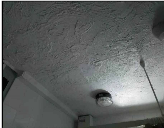
Ground Floor Bathroom (G.001) Textured Coating/Paint Ceiling,
