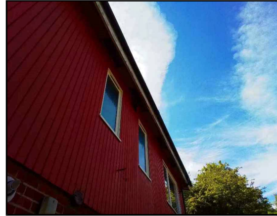
External External (E.001) Cement Products Soffits,
