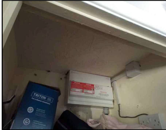
Ground Floor Cupboard - Store (G.005) Textured Coating/Paint Ceiling,
