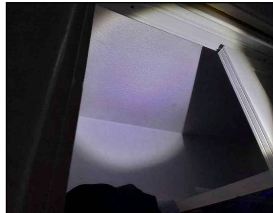
1st Floor Bedroom 3 (1.005) Textured Coating/Paint Ceiling, Within cupboard
