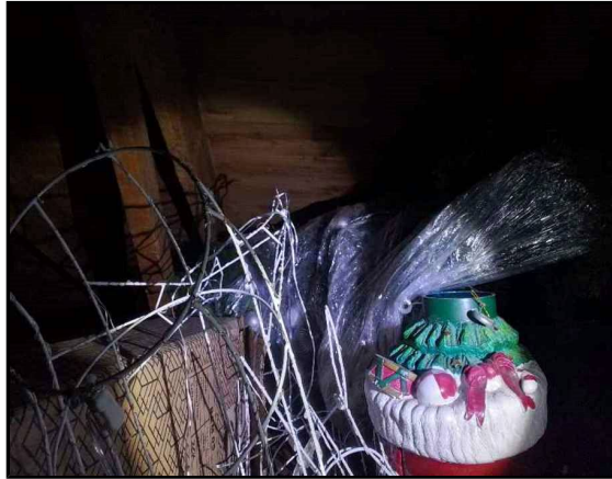
Roof Void Loft Space (R.001) Inaccessible Roof
