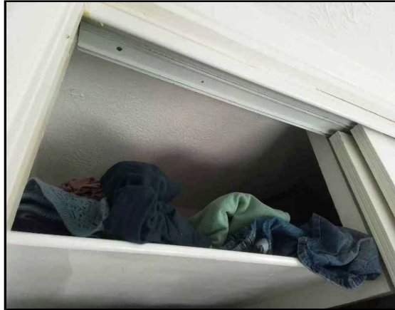
1st Floor Bedroom 1 (1.001) Textured Coating/Paint Ceiling, Within cupboard
