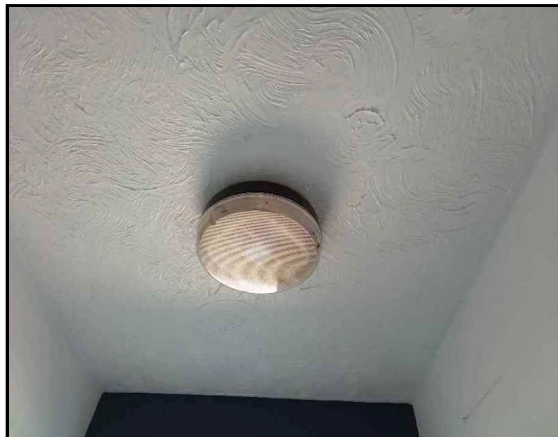
1st Floor Bathroom (1.004) Textured Coating/Paint Ceiling,
