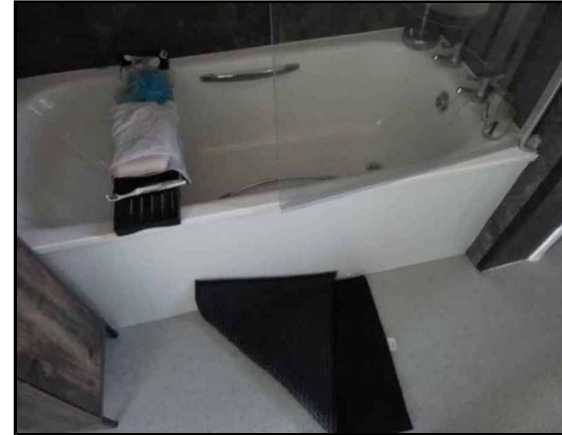
1st Floor Bathroom (1.003) Inaccessible Bath Panel No access behind plastic bath panel
