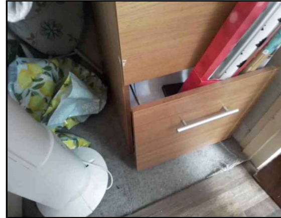
Ground Floor Cupboard - Store (G.005) Composite Vinyl Tile, Vinyl/Lino with adhesive Floor,
