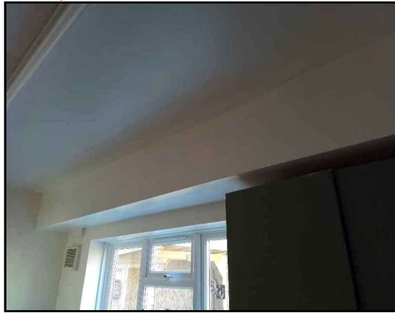
Ground Floor Kitchen (G.003) Inaccessible Bulkhead No access within sealed boxing
