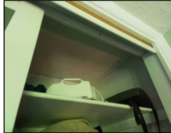
1st Floor Bedroom 2 (1.002) Textured Coating/Paint Ceiling, Within cupboard
