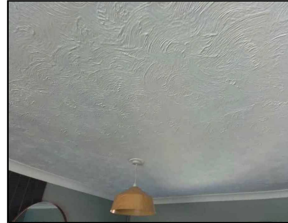
Ground Floor Living Room/Lounge (G.006) Textured Coating/Paint Ceiling,
