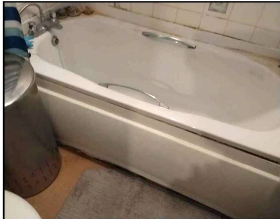
Ground Floor Bathroom (G.002) Inaccessible No access behind bath panel
