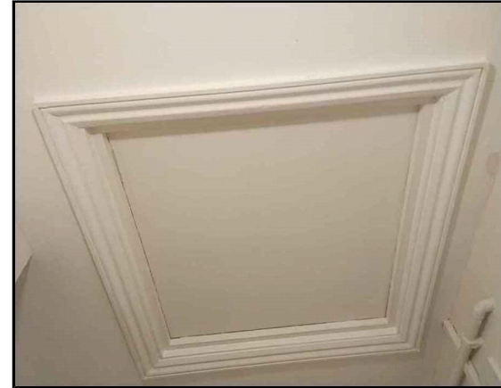
Roof Void Loft Space (R.001) Inaccessible
