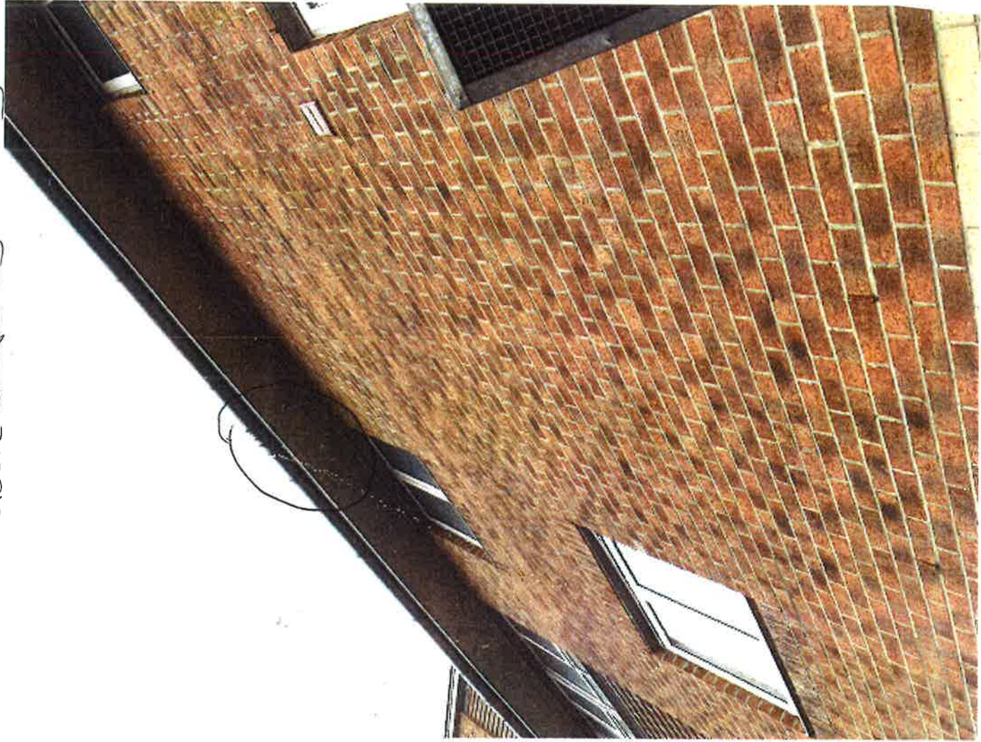
Side of building by laundry above steps by laundry room exit
