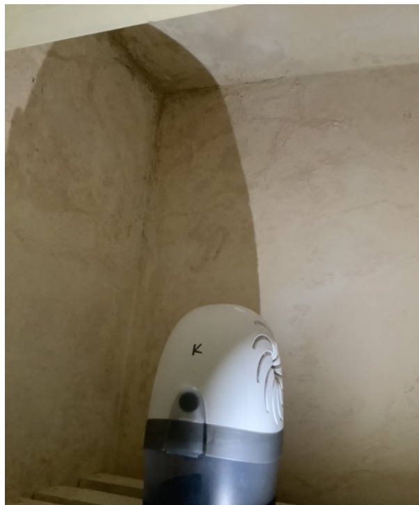
Image of mould growth and damp penetration to storage cupboard
