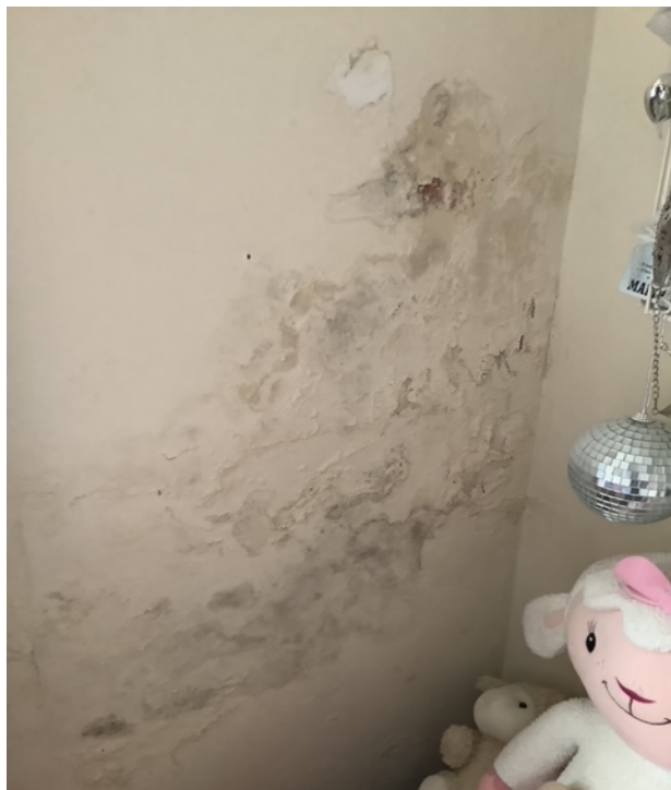
Image of damp penetration to rear wall of bedroom
