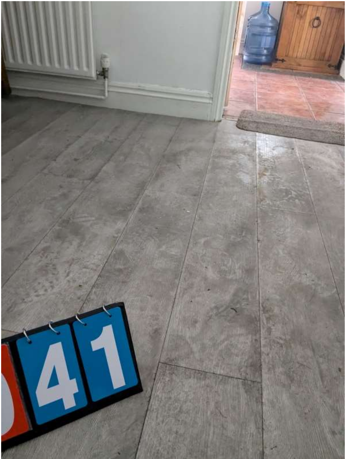
0041 – Water damage/cupping to dining room laminate flooring. 21/8/24 95
