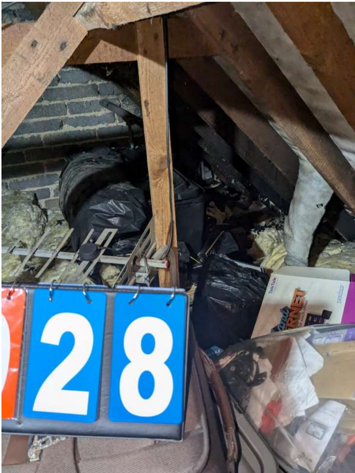
0028 – Loft, fire damage visible to rafters. 19/8/24
