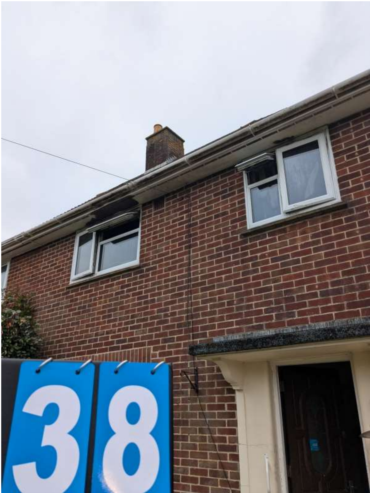
0038 – Front Elevation, damage to soffit/facia. 19/8/24
