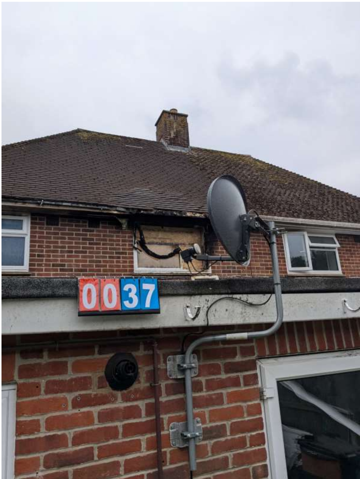
0037 – Rear elevation, fire damage to Bedroom 1 window and roof. 19/8/24
