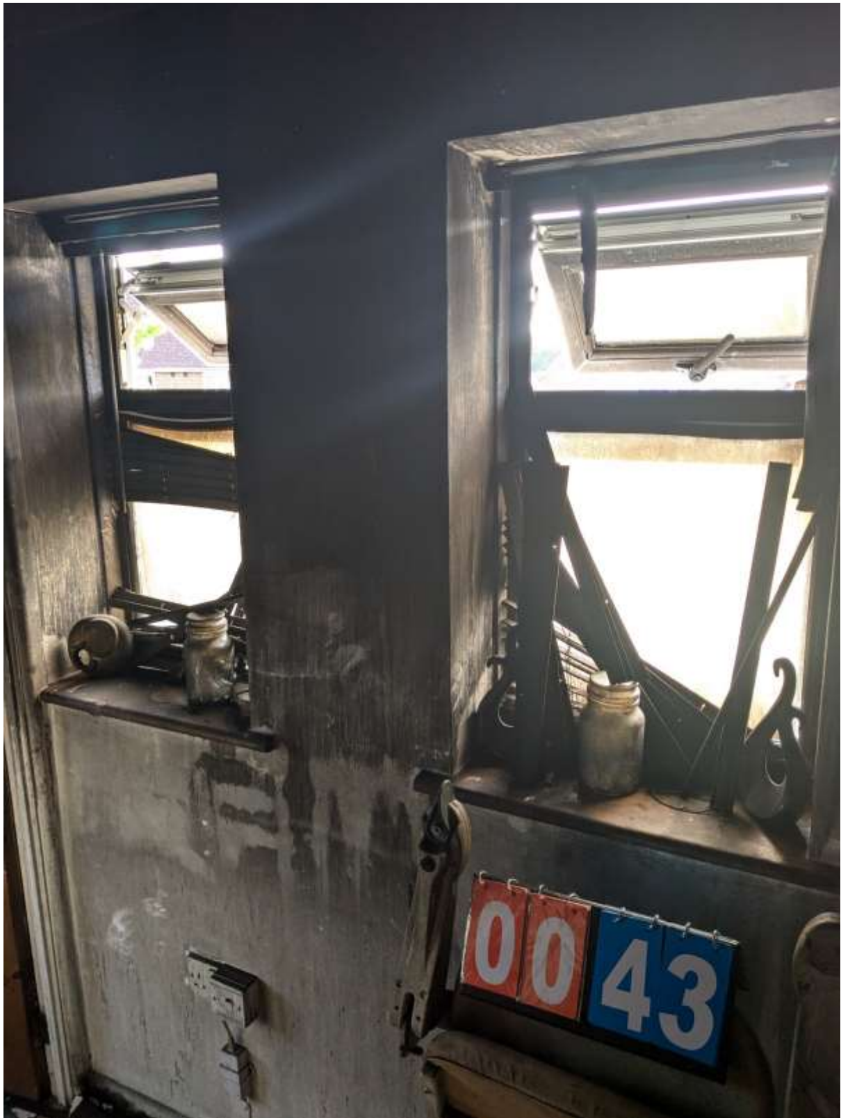
0043 – Fire/smoke damage to 1 st floor hallway windows. 21/8/24 97
