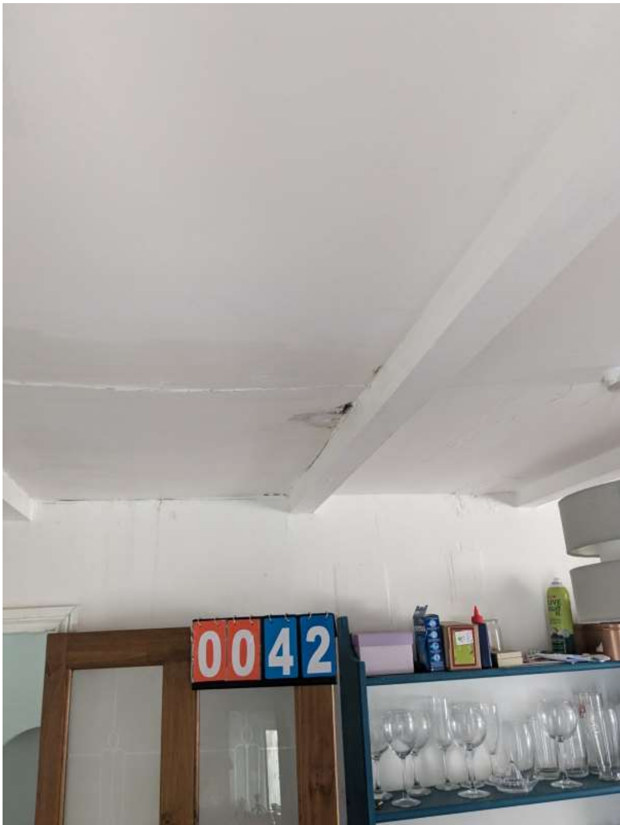
0042 – Water damage to kitchen hallway ceiling. 21/8/24
