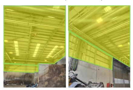
The netting will be attached to 2mm stainless steel wire tailored to fit as flush as possible under the vents and cable trays. The lighting will require access zips in the netting for servicing to be possible when required.
